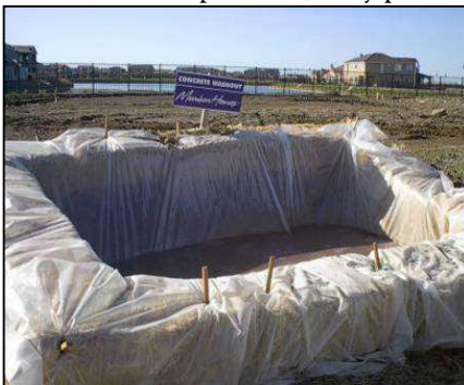
Plate 3-1 Typical concrete shoot wash out areas
