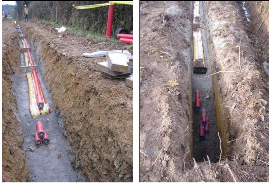
Plate 2-1 Cable Trench View
